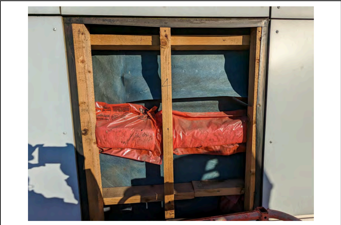
Photo 11: Location 4 - HPL removed on 3rd floor at front facade
