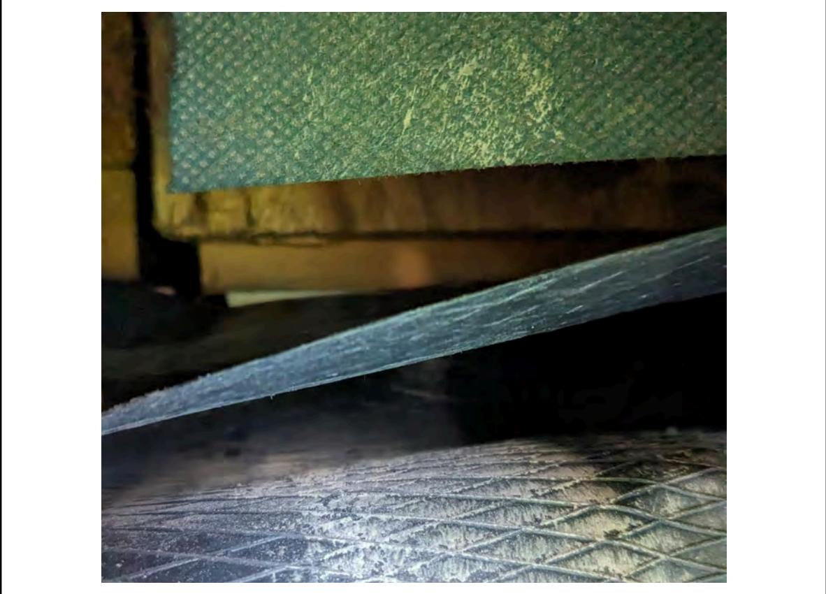
Photo 62: Location 29 - Brick build up
