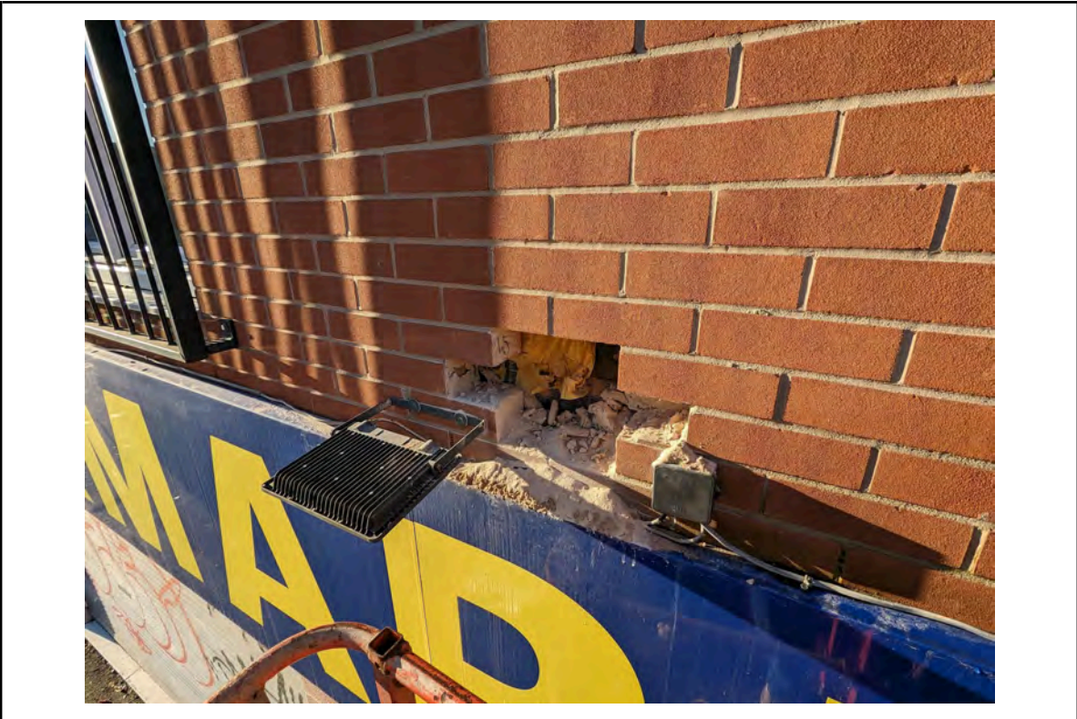
Photo 33: Location 15 - Brick removed on 1st floor at east elevation
