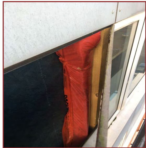
Images showing the horizontal and vertical Rockwool 'sock' fire barriers. Their fitting, which doesn't cover the entire cavity, means that they will not be able to perform their task effectively.
