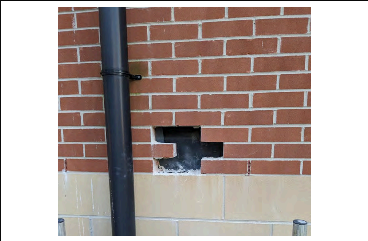
Photo 61: Location 29 - Brick removed at 1st floor at courtyard elevation
