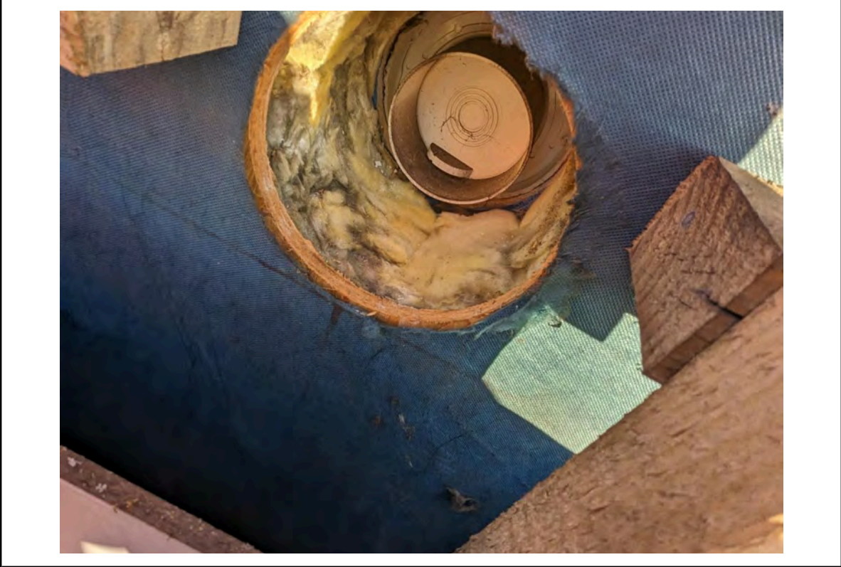
Photo 18: Location 7 - HPL facade build up
