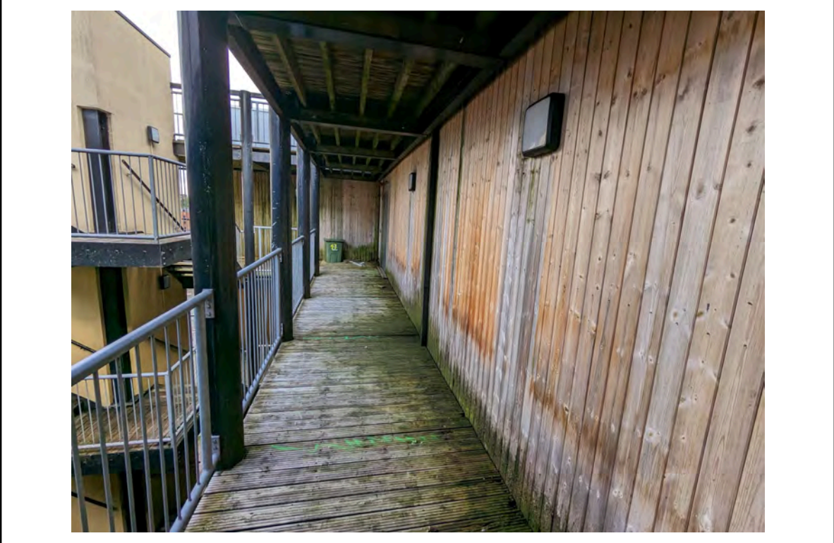
Photo 66: General view of exterior walkway at inner courtyard area
