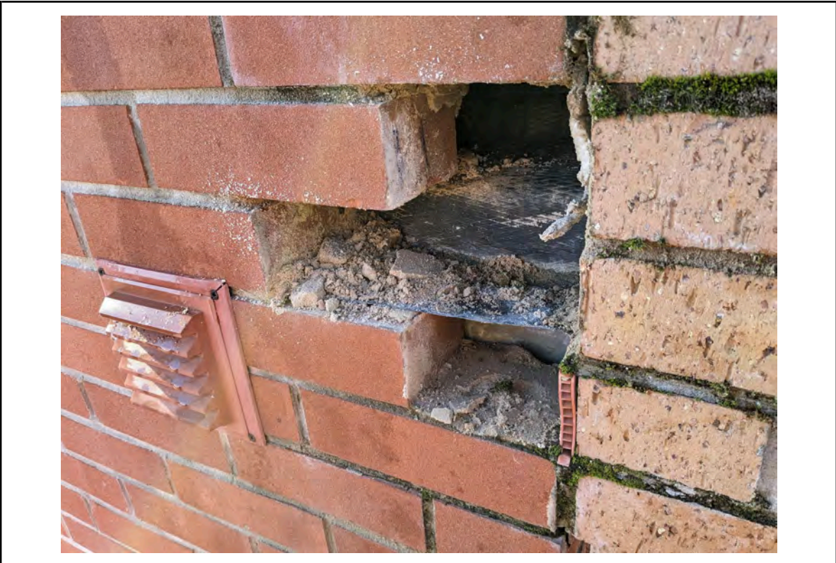
Photo 25: Location 11 - Brick removed on 2nd floor at east elevation
