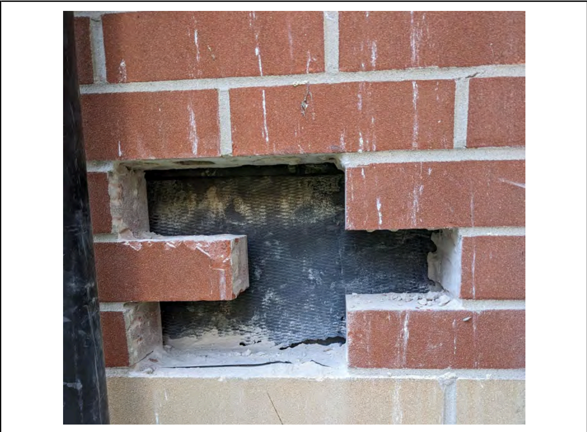
Photo 63: Location 30 - Brick removed at 1st floor at courtyard elevation
