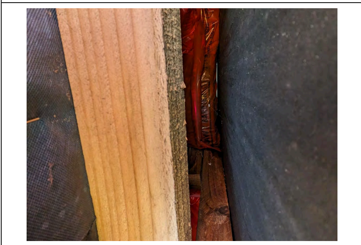
Photo 14: Location 5 - Cavity of cavity barrier, breather membrane and timber studs
