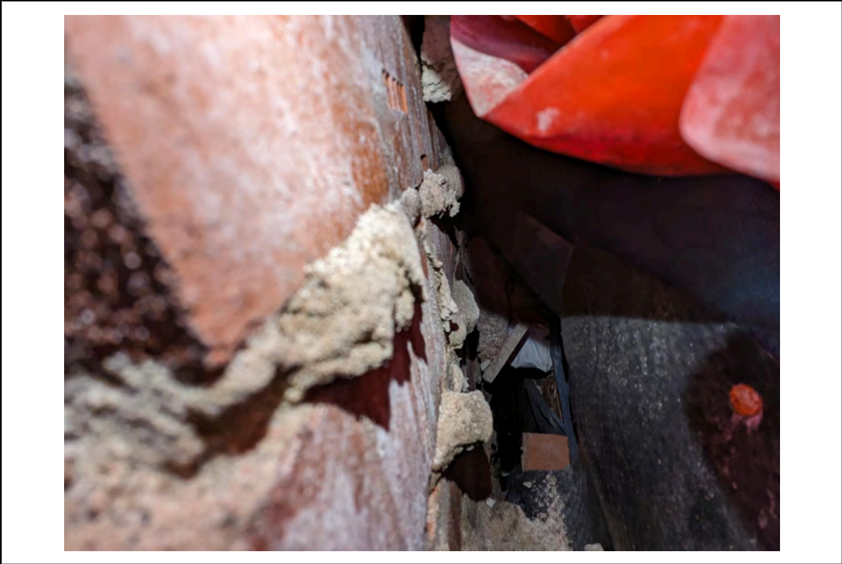
Photo 16: Location 6 - Cavity with damp proof membrane, breather membrane and cavity barriers
