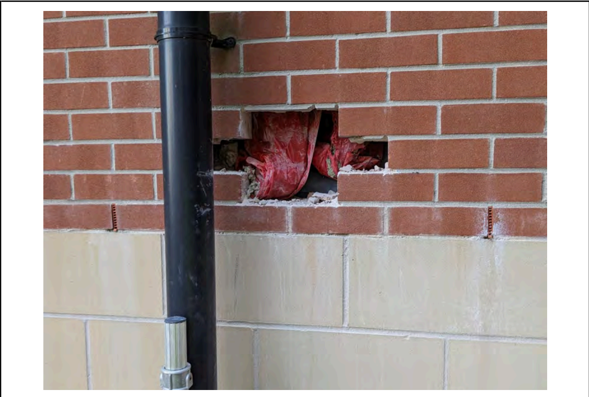
Photo 43: Location 20 - Brick removed on 1st floor at courtyard elevation
