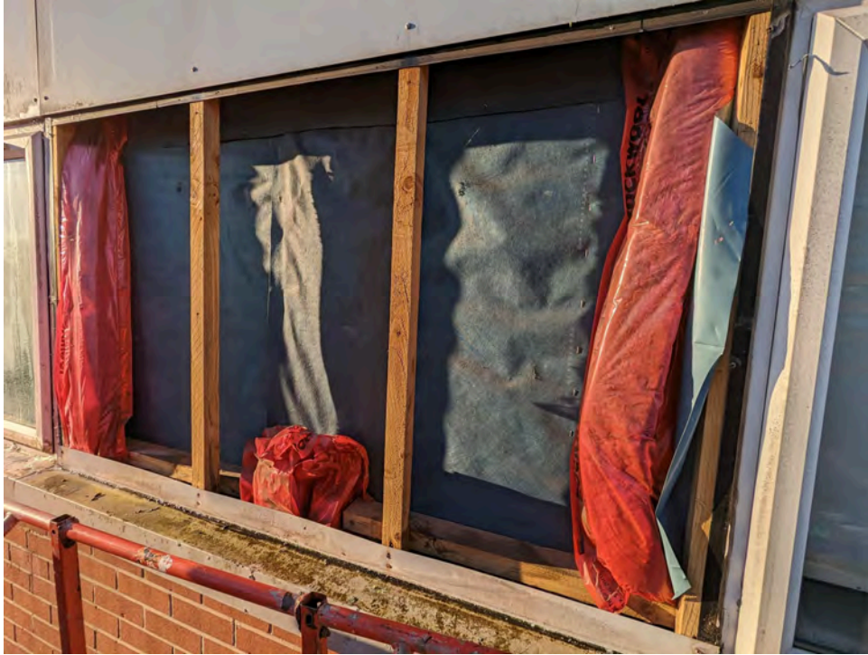
Photo 35: Location 16 - HPL removed on 3rd floor at east elevation
