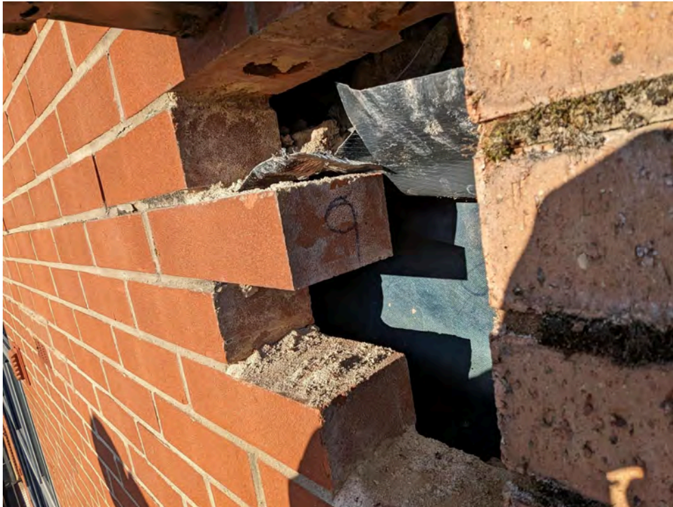
Photo 21: Location 9 - Brick removed on 2nd floor at south elevation
