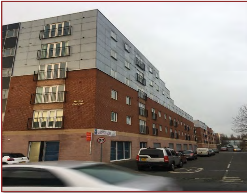
South East Elevation showing roller shutter doors to the ground floor commercial space. There are windows to each flat, some with Juliette balconies whilst the top three floors are covered with a cladding material.
