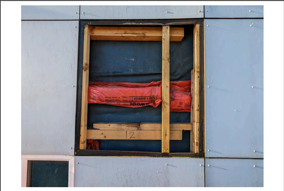
Photo 27: Location 12 - HPL removed on 3rd floor at east elevation
