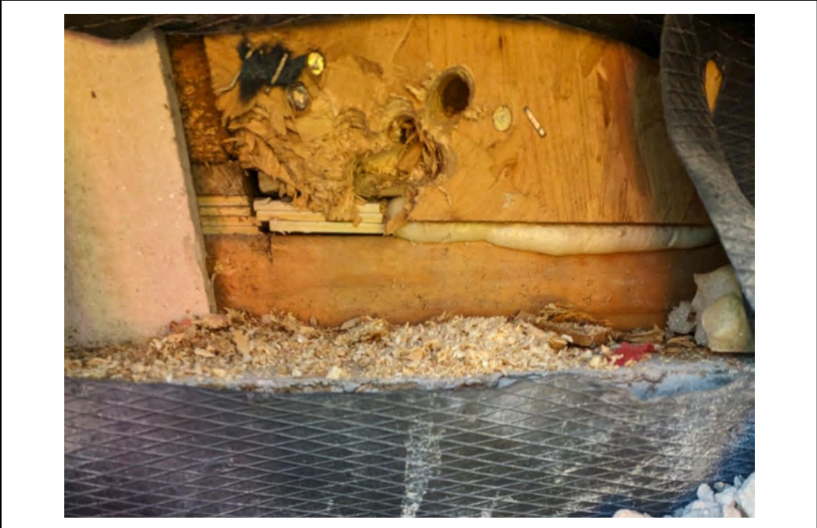
Photo 34: Location 15 - Cavity with damp proof membrane, breather membrane and timber frame
