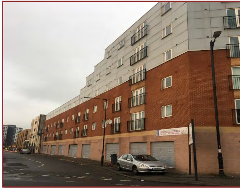
South West Elevation showing roller shutter doors to the ground floor commercial space. There are windows to each flat, some with Juliette balconies whilst the top three floors are covered with a cladding material.
