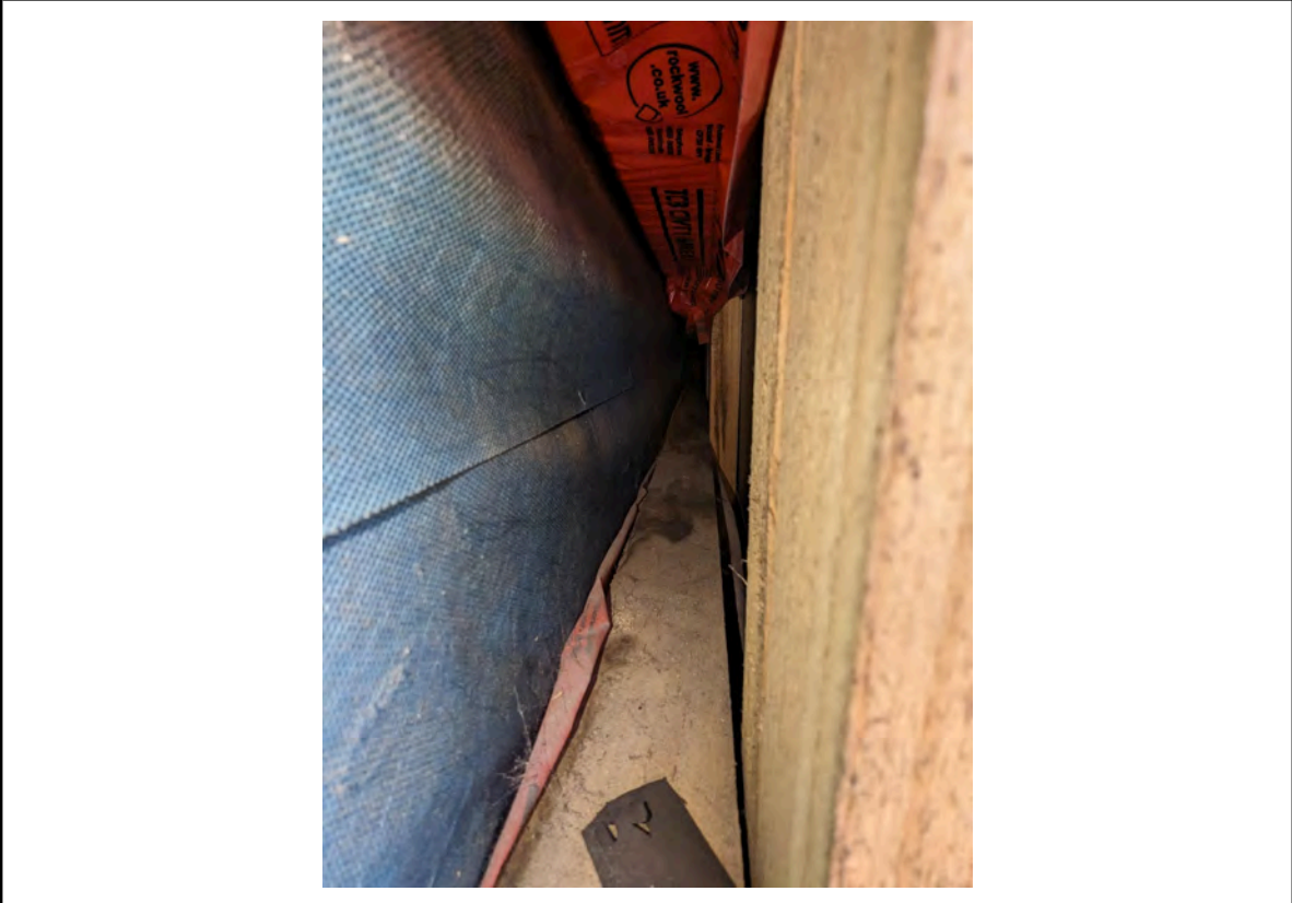
Photo 12: Location 4 - Cavity showing timber studs, breather membrane and cavity barriers
