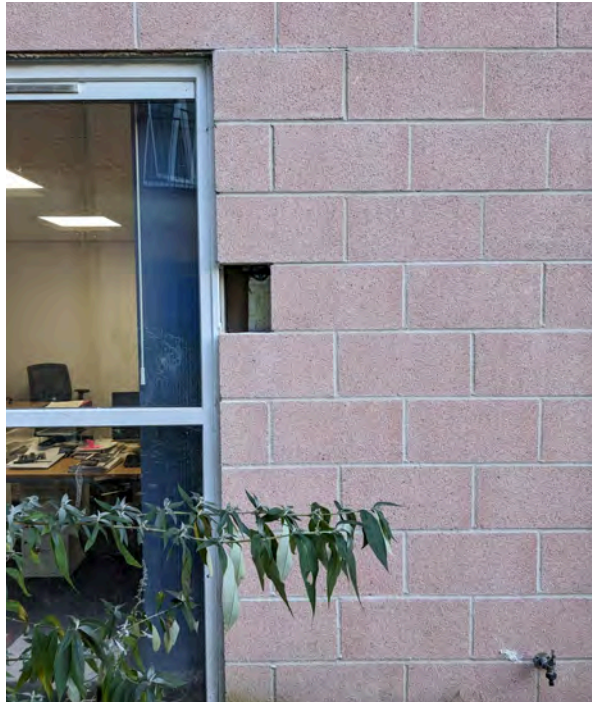
Photo 57: Location 27 - Artstone removed at ground floor at courtyard elevation
