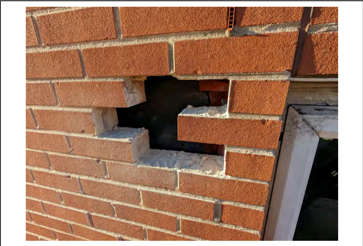
Photo 31: Location 14 - Brick removed on 2nd floor at east elevation
