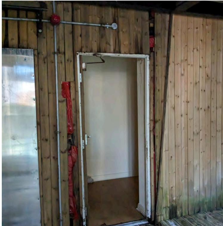
Photo 45: Location 21 - Timber cladding removed on 2nd floor at inner courtyard elevation
