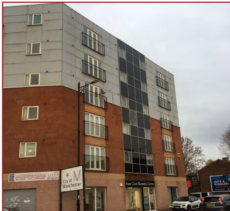
South Elevation with curtain walling to the ground floor commercial space and ground to floor feature area, windows to each flat with Juliette balconies. The top three floors are covered with a cladding material.
