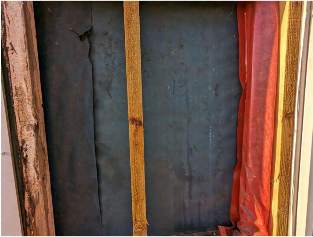
Photo 29: Location 13 - HPL removed on 2nd floor at east elevation
