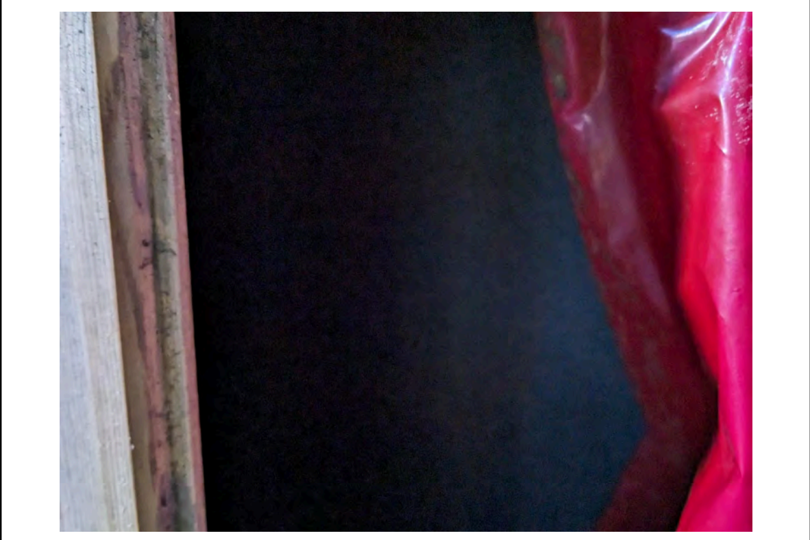
Photo 50: Location 23 - Cavity showing cavity closer at window openings and breather membrane
