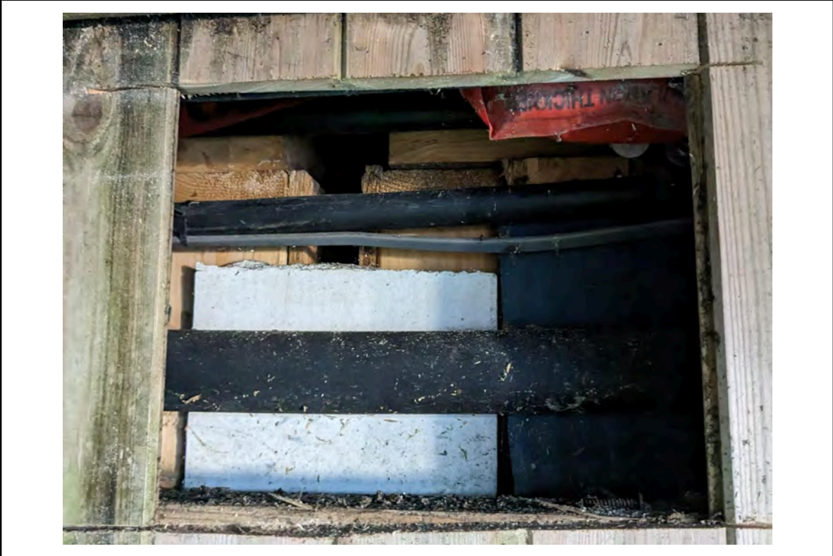
Photo 48: Location 22 - Timber cladding system build up
