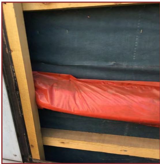
Images showing the horizontal and vertical Rockwool 'sock' fire barriers. Their fitting, which doesn't cover the entire cavity, means that they will not be able to perform their task effectively.
