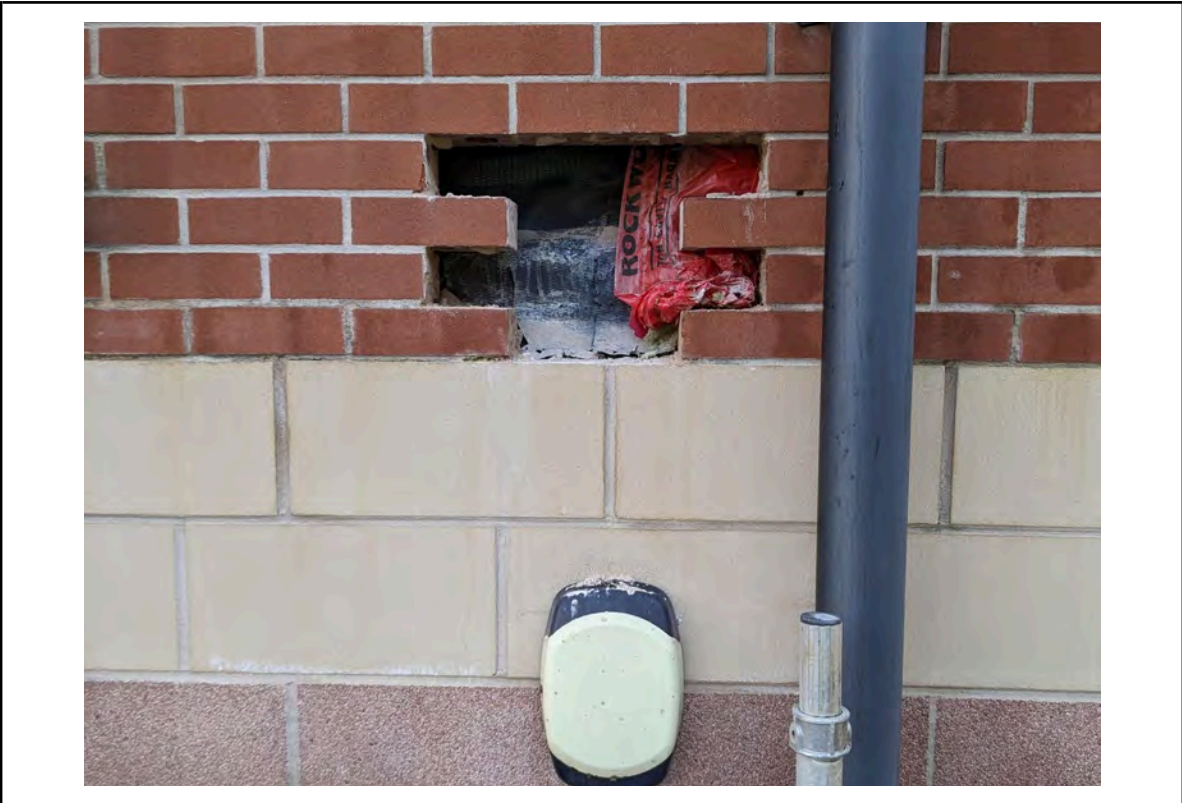
Photo 39: Location 18 - Brick removed on 1st floor at courtyard elevation
