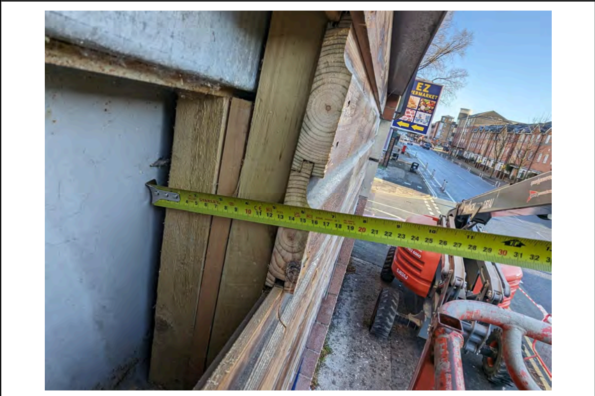
Photo 24: Location 10 - timber spandrel panel build up
