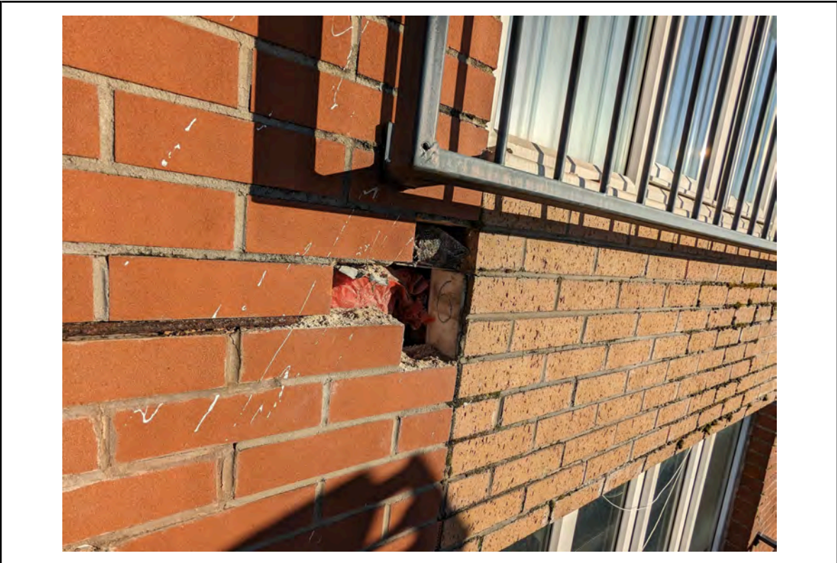
Photo 15: Location 6 - Brick removed on 2nd floor at front facade
