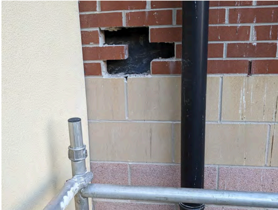
Photo 59: Location 28 - Brick removed at 1st floor at courtyard elevation
