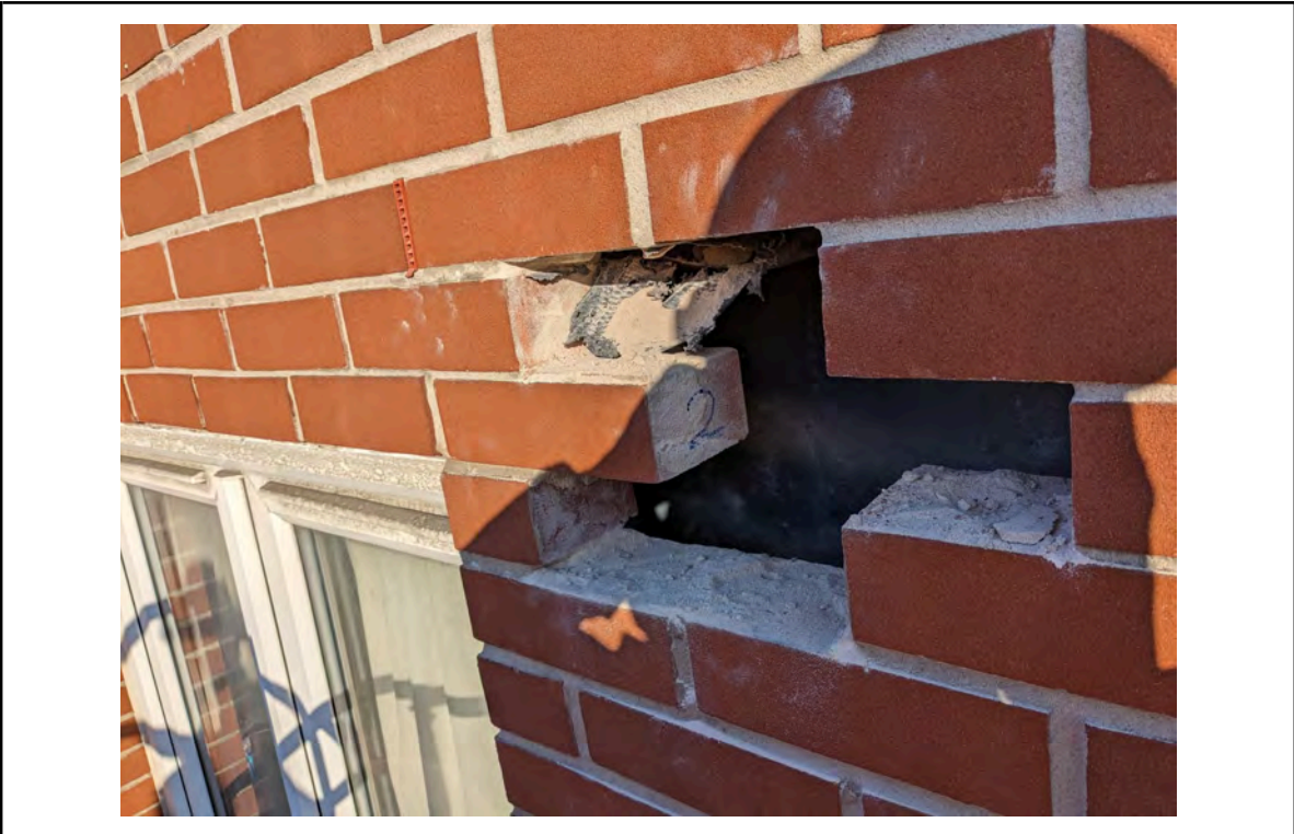
Photo 7: Location 2 - Brick removed on 1st floor at front facade
