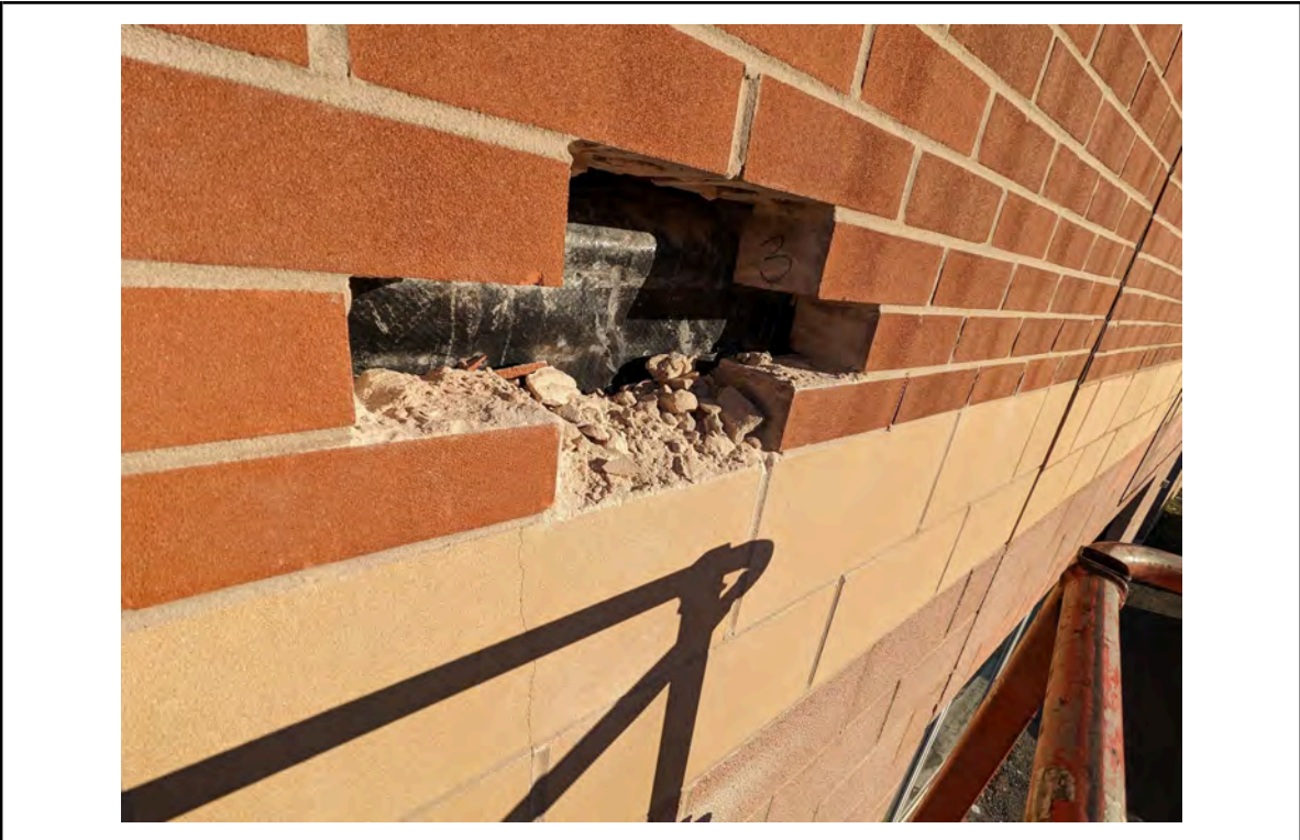
Photo 9: Location 3 - Brick removed on 1st floor at front facade
