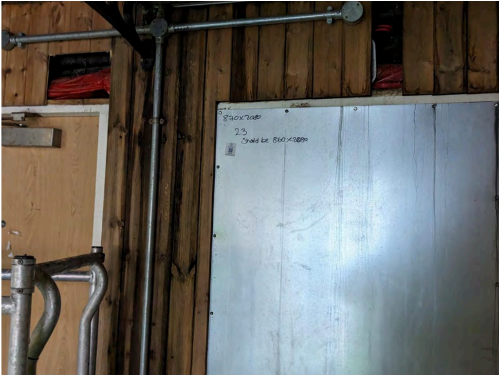
Photo 55: Location 26 - Timber cladding removed on 2nd floor at inner courtyard elevation
