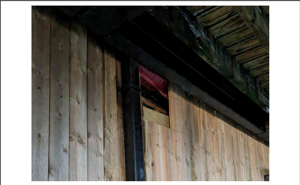
Photo 47: Location 22 - Timber cladding removed on 3rd floor at inner courtyard elevation
