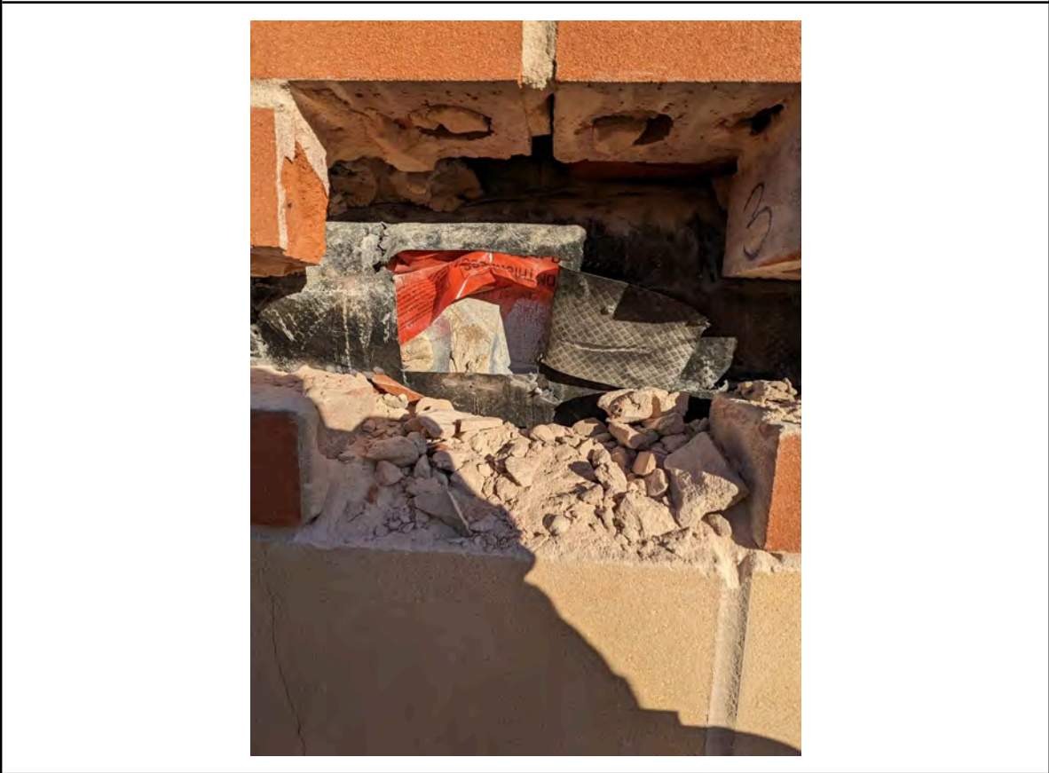
Photo 10: Location 3 - Cavity with wall ties, damp proof membrane and cavity barriers
